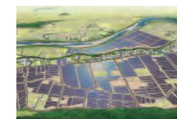
Mega Solar Power Plant in Yatsuda District of Namie Town
