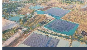
Floating Solar PV, TSB Co., Ltd., Thailand
